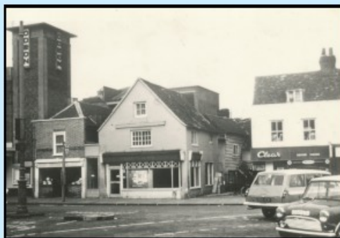
View of High Street site before demolition in 1969. No. 110 is the larger building, gable-end to the street
